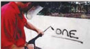
Graffiti cleaning contractor
